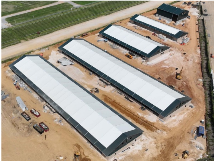
Backstretch buildings: Laying the groundwork brick by brick along the Pimlico backstretch. Masonry, building envelope, and MEP systems are moving full speed ahead!
